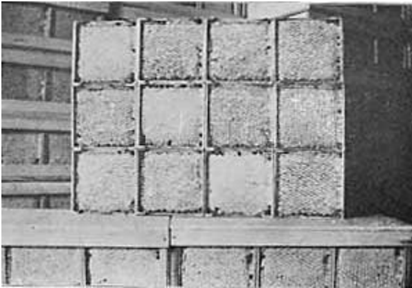
Fig. 100—Sections Ready for Casing.
